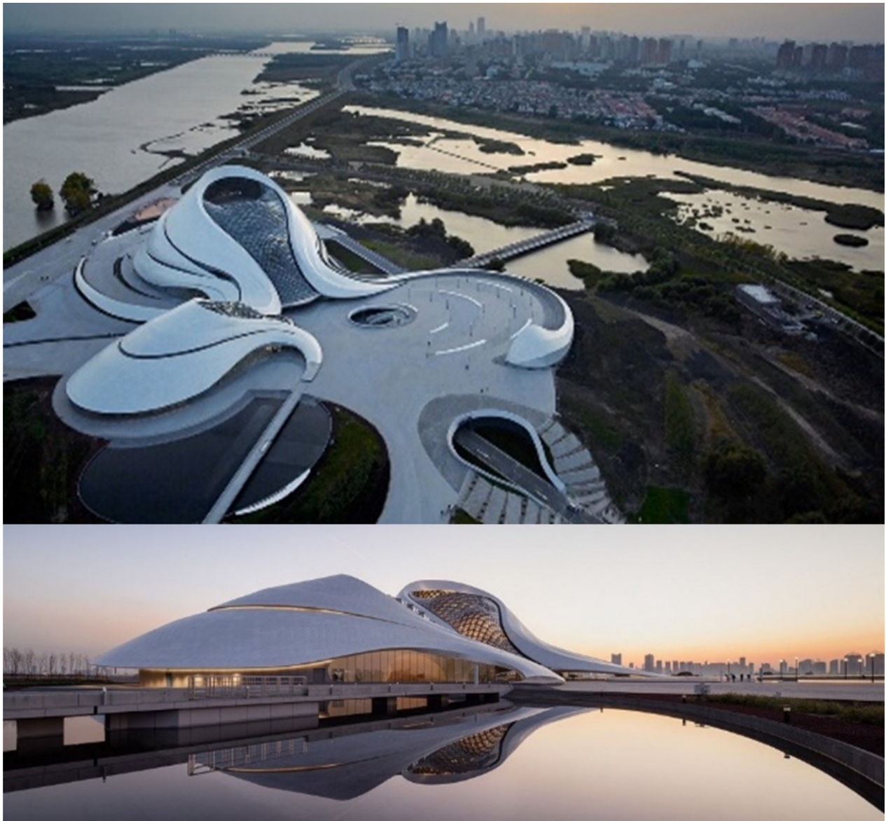
Picture 2. Harbin Opera House. MAD Architects
