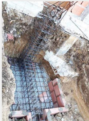
Figure 3.12 – Cantilever or strip foundation
