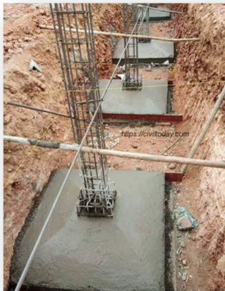
Figure 3.11 – Isolated shallow foundation
