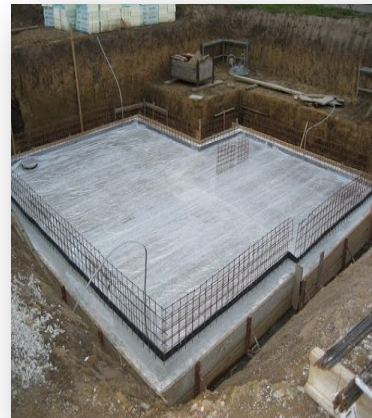
Figure 3.13 – Raft or pad foundations
