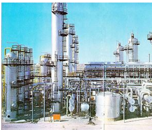
Oil refinery in Iran.
