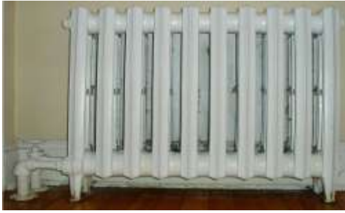
A cast iron household radiator.
